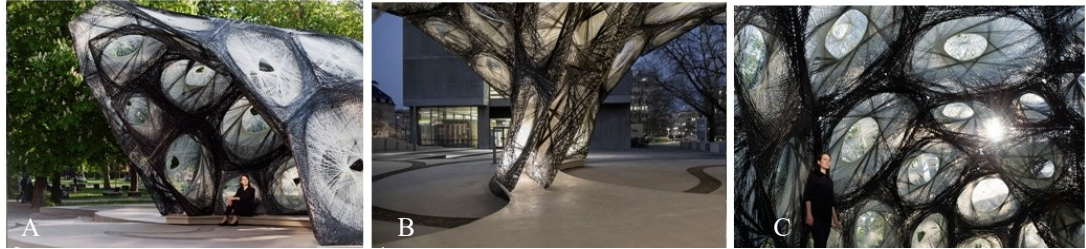
Figure 4.18: Pavilion ( A: Overhang image, B: Interior image, C: Component system) (Dörstelmann et al., 2014, p. 227)
