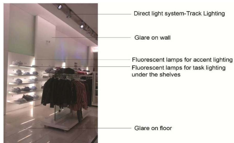
Figure 5.8: A view from the casual department and its features- Coordinates on plan B19
