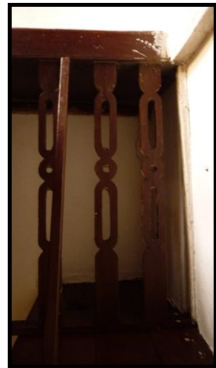
Figure 112: Detail from handrail in 11-Hamam Street
