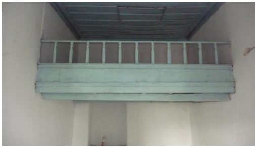
Figure 86: Storage unit above the staircase in 39-Türkkuyusu Street
