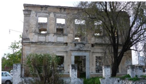
Figure 50: Front view of Kocadon House
