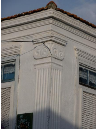
Figure 62: Column and capital detail from 60-Türkkuyusu Street
