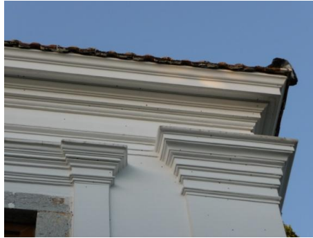
Figure 35: Cornice and capital detail from 50-Türkkuyusu Street
