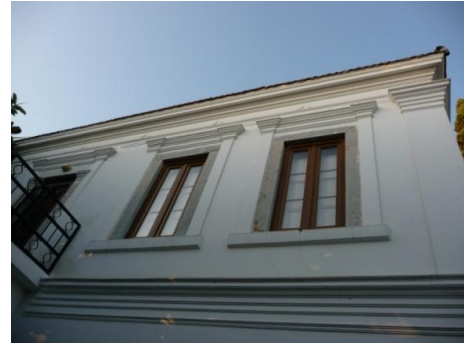
Figure 36: Window, cornice and column detail from 50-Türkkuyusu Street
