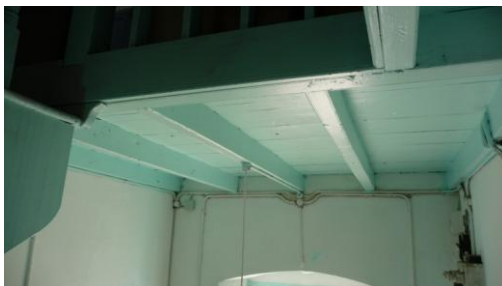
Figure 153: Detail of the slab from 1-Artemis Street
