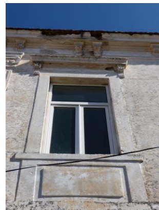
Figure 49: Window frame detail from 32-Çukurbahçe Street
