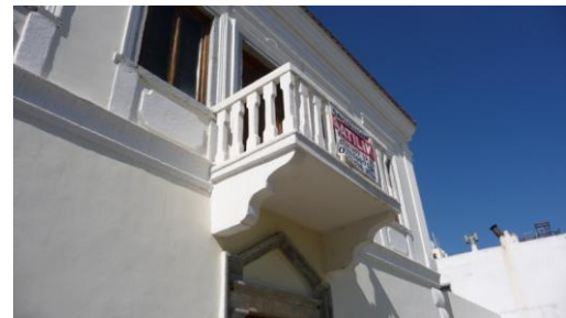
Figure 32: The Balcony of 29-Atatürk Street
