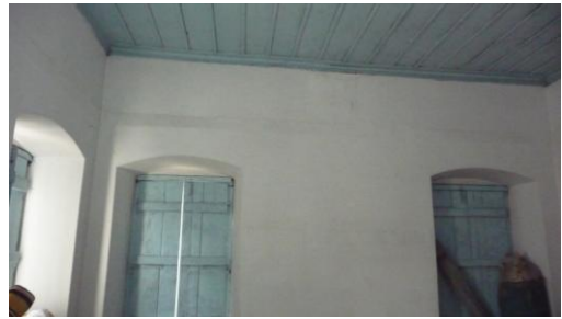
Figure 87: An interior view from the first floor of 39-Türkkuyusu Street
