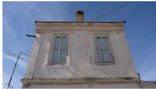
Figure 125: Left view of 19-Hamam Street
