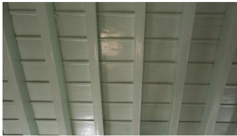
Figure 130: Ceiling of ground floor of 19-Hamam Street
