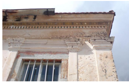
Figure 75: Window frame, cornice, column and capital of 39-Türkkuyusu Street
