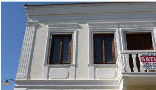
Figure 31: Window, cornice and column details from 29-Atatürk Street
