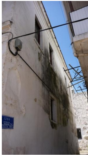
Figure 101: Rear view of 11-Hamam Street
