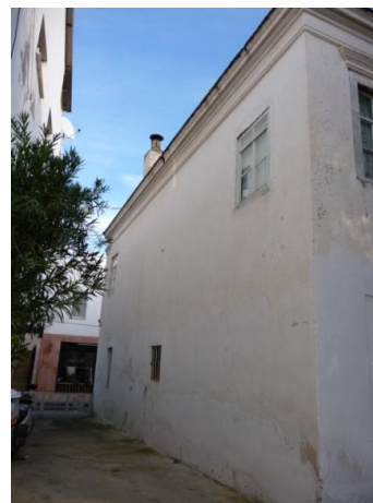
Figure 73: Rear-Right view of 39-Türkkuyusu Street
