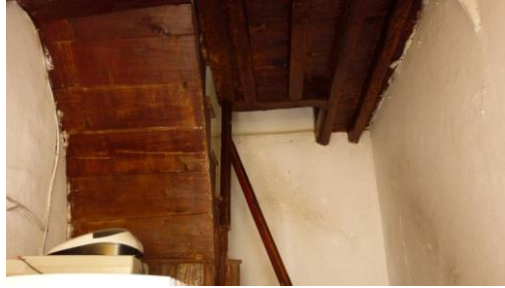
Figure 110: Staircase of 11-Hamam Street
