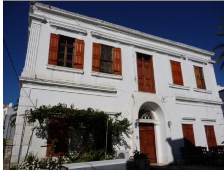
Figure 37: Front view of 20-Neyzen Tevfik Street
