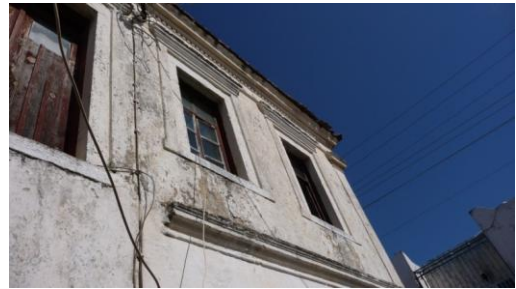
Figure 98: An exterior view of 11-Hamam Street
