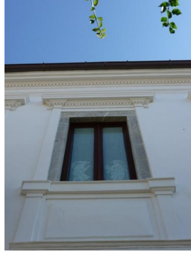
Figure 60: Window and window frame detail from 141-Cumhuriyet Street
