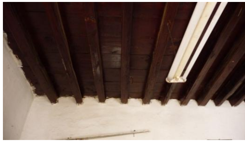
Figure 108: Ground floor ceiling of 11-Hamam Street
