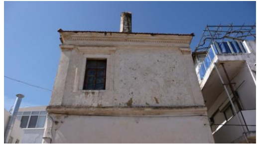
Figure 100: Left view of 11-Hamam Street
