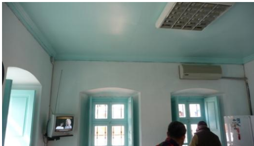
Figure 151: An interior view from the ground floor of 1-Artemis Street
