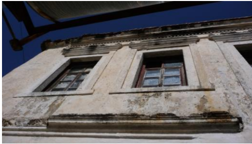
Figure 99: An exterior view of 11-Hamam Street
