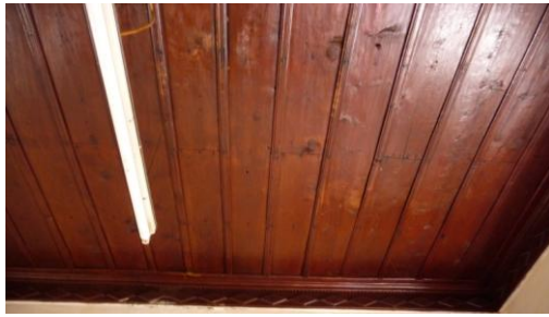
Figure 113: Ceiling of the first floor in 11-Hamam Street
