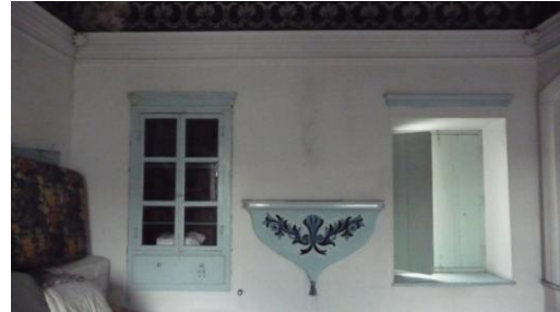
Figure 83: An interior view from the first floor of 39-Türkkuyusu Street
