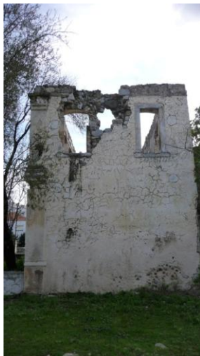
Figure 52: Left view of Kocadon House
