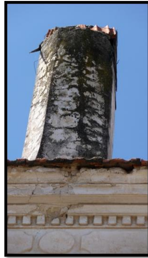
Figure 102: Chimney of 11-Hamam Street
