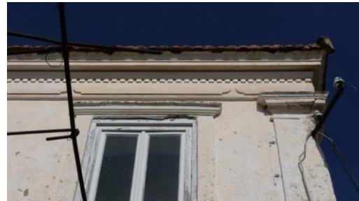
Figure 127: Window frame, cornice and capital detail from 19-Hamam Street
