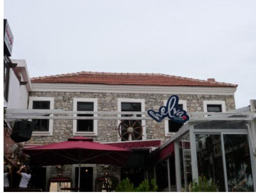
Figure 68: Front view of 44-Neyzen Tevfik street
