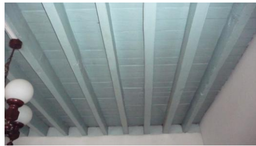
Figure 77: Ceiling of ground floor of 39-Türkkuyusu Street
