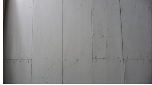
Figure 135: Floor finishing of the first floor of 19-Hamam Street
