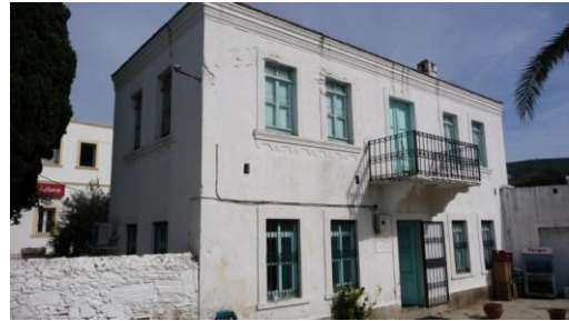
Figure 146: Front-Right view of 1-Artemis Street
