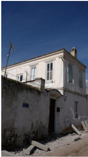
Figure 124: Front-Left view of 19-Hamam Street
