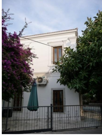
Figure 33: Right view of 50-Türkkuyusu Street
