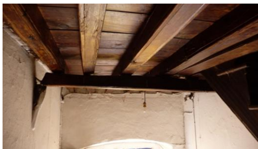
Figure 111: Slab detail from 11-Hamam Street
