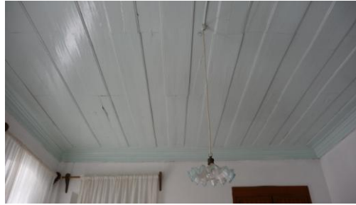
Figure 136: Ceiling of the first floor of 19-Hamam Street
