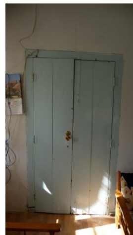
Figure 133: Interior door in the ground floor of 19-Hamam Street
