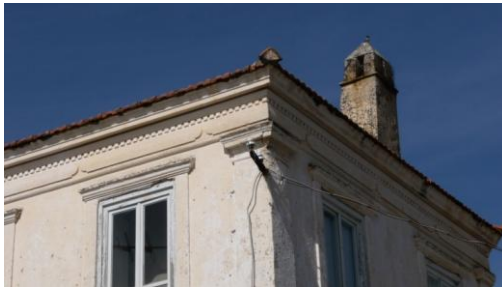
Figure 126: An exterior view of 19-Hamam Street
