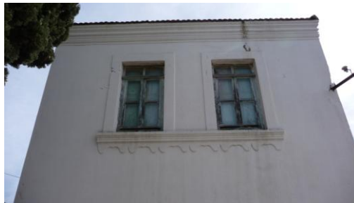
Figure 147: Right view of 1-Artemis Street
