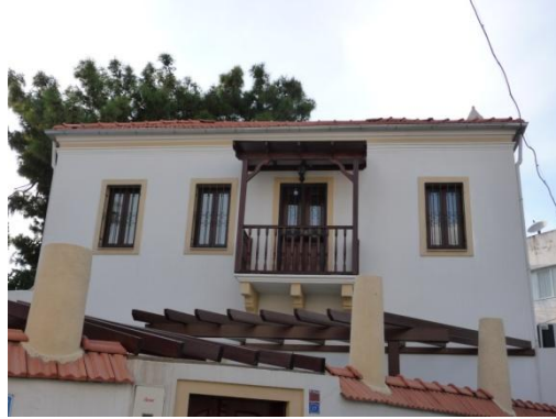
Figure 66: Front view of 17-Gerence Street
