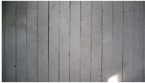
Figure 155: Floor finishing of the first floor of 1-Artemis Street
