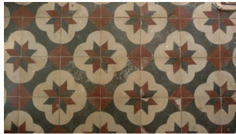
Figure 131: Floor finishing in the entrance of 19-Hamam Street
