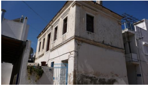
Figure 97: Front-Left View of 11-Hamam Street
