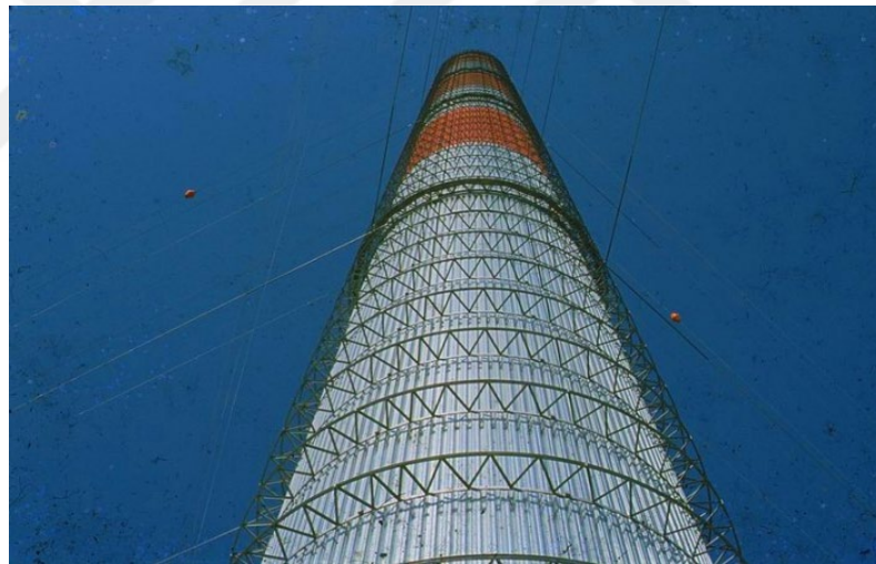
Figure 1.6: The tower structure of SCPP [11].
