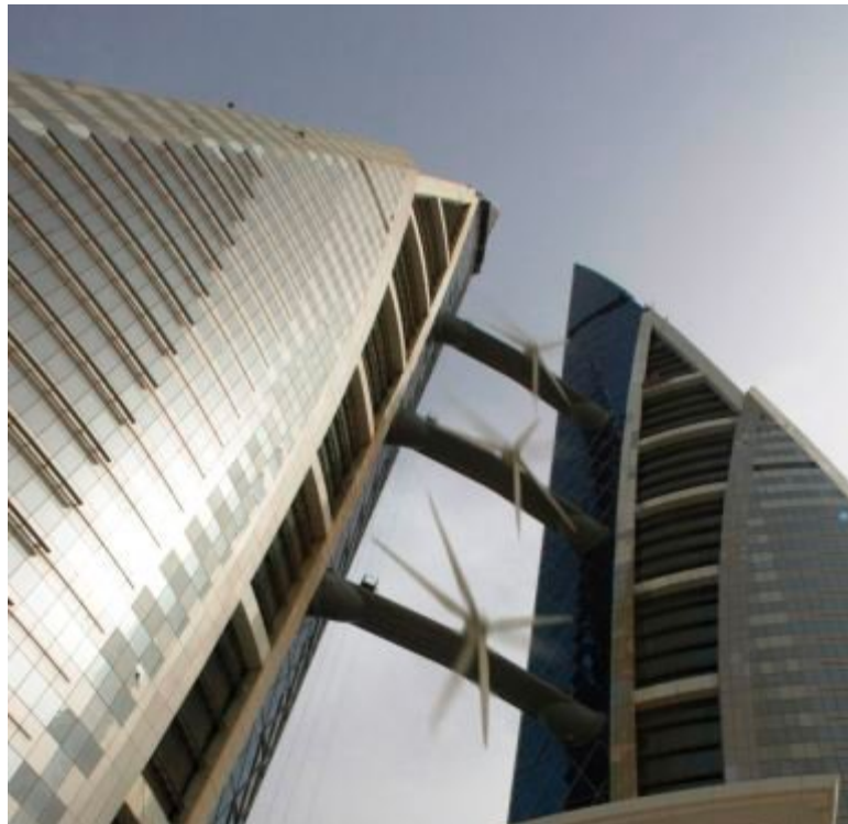
Figure 3.2: Wind turbines in Bahrain World Trade Center, Bahrain
