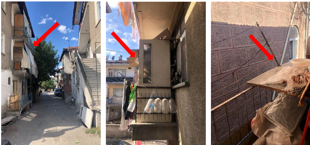
Figure 66: Coverings of the Balconies in the Sample (Author, 2019).
