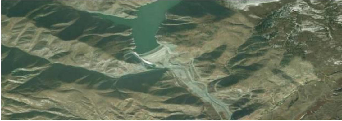
Figure 40 Top view of Karadere Dam and its lake, in Kastamonu Province
