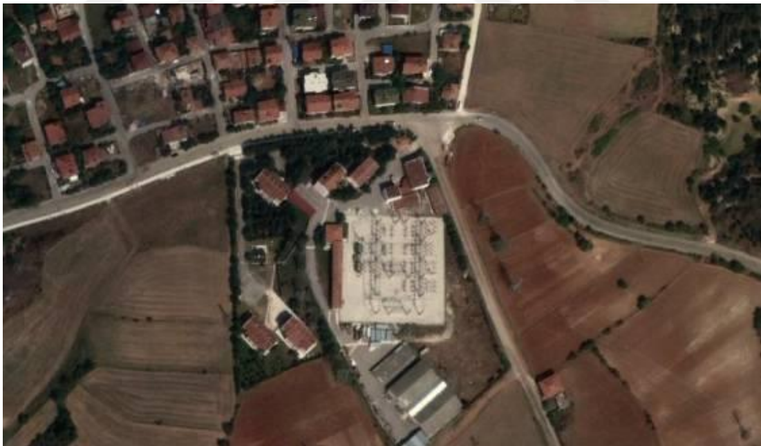
Figure 71 Top view of Kastamonu Substation
