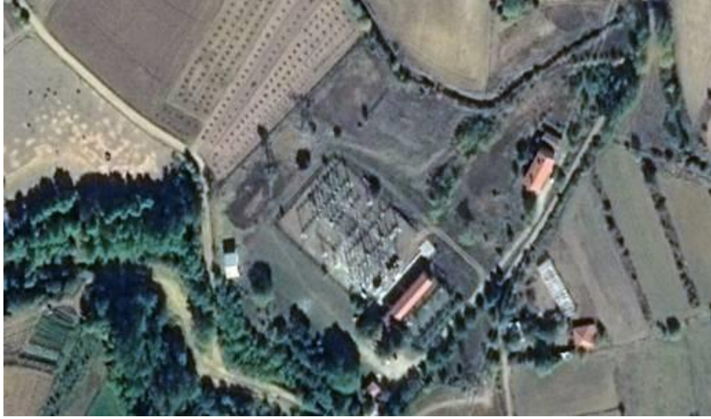
Figure 43 Top view of Taşköprü Substation
