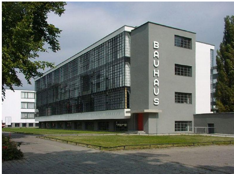
Figure 27 The Bauhaus building, Walter Gropius, 1926
