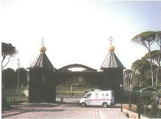
Figure 4-13 View from the interior towards the Main Entrance Door of VPRH, 2003.
