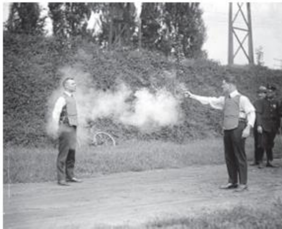
Figure 3 Bulletproof vest test in 1923 [1]
