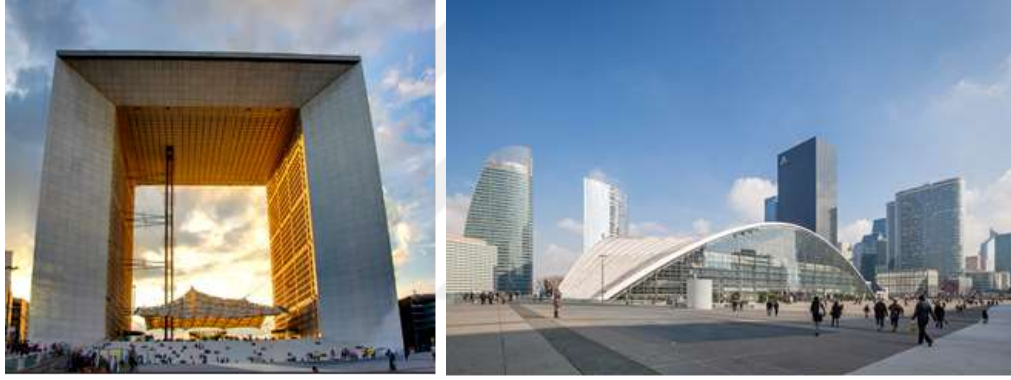
Şekil 2. 30: Grande Arche (url-54), Le Centre National de Industries et Techniques (url-55)
