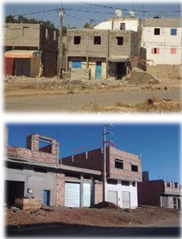
Figure 4: Kirkuk has experienced a considerable increase in illegal slums
