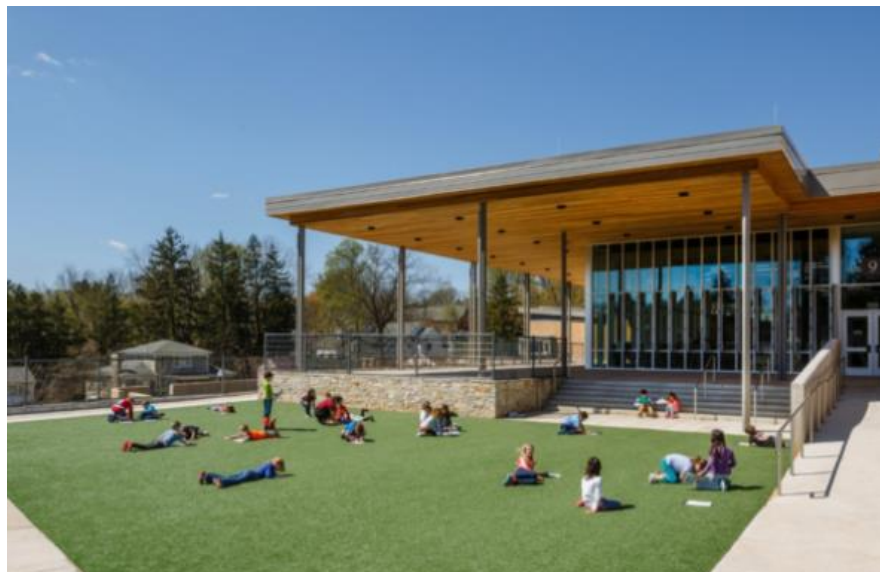
Figure 59: Discovery Elementary School / USA (URL-26)
