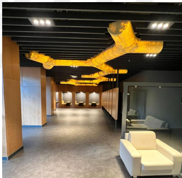
Figure 90: The forms on the ceiling tiles are suitable for biomorphic patterns in Common Area Used by Faculty of Architecture and Faculty of Law (Parameter 8) (Author's Archive)
