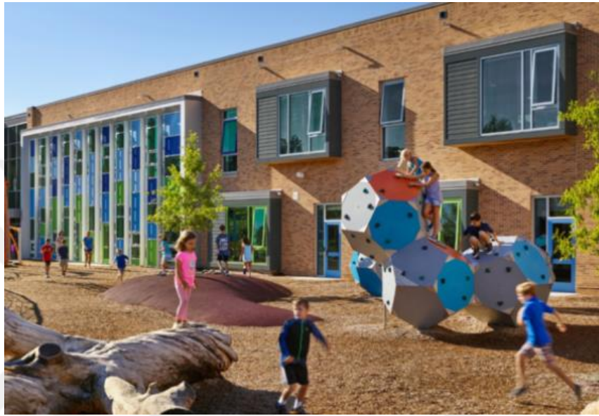
Figure 60: Discovery Elementary School / USA (URL-26)
