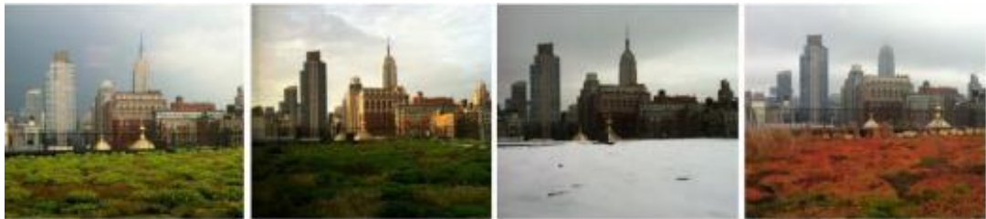
Figure 19 : Green roof of Cookfox Architects' building, New York, USA (Browning 2014: 27).
