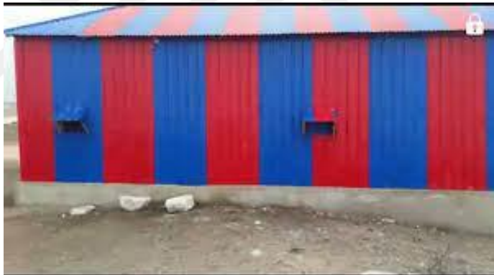
Figure 3.28: House made of corrugated iron sheet (ba'awayne) in the outskirts of mogadishu source from suuqfudud (Facebook Gal | Facebook-Ga, n.d.)
