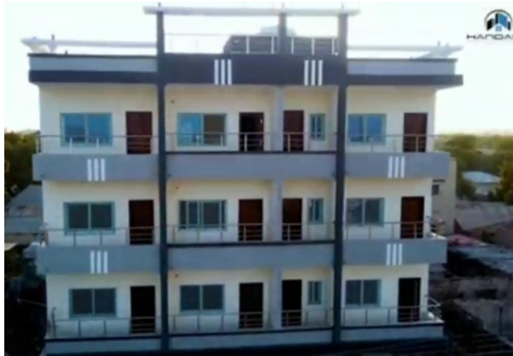
Figure 3.36: Front view of apartment 1 (source owner)
