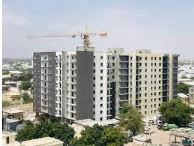
Figure 3.33: MOGADISHU | Sunrise Apartments | Under construction (MOGADISHU | Sunrise Apartments | U/C | SkyscraperCity Forum, 2008)
