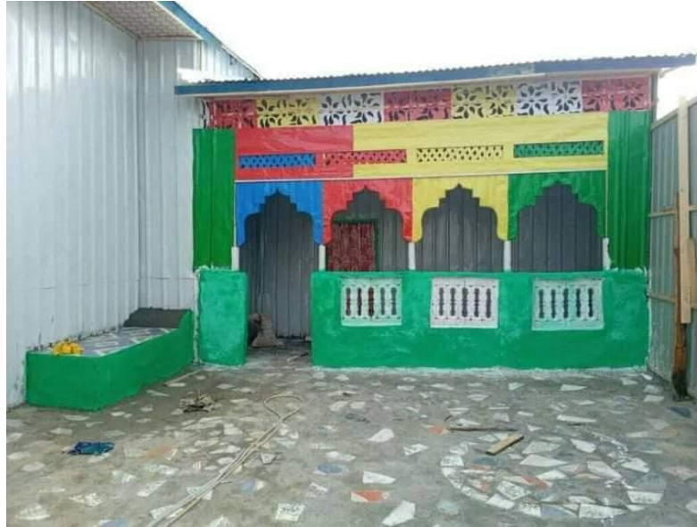
Figure 3.29: House made of corrugated iron sheet (ba'aweyne) in the outskirts of mogadishu (Dhulkoob - Powerful Residence Real Estate, n.d.)
