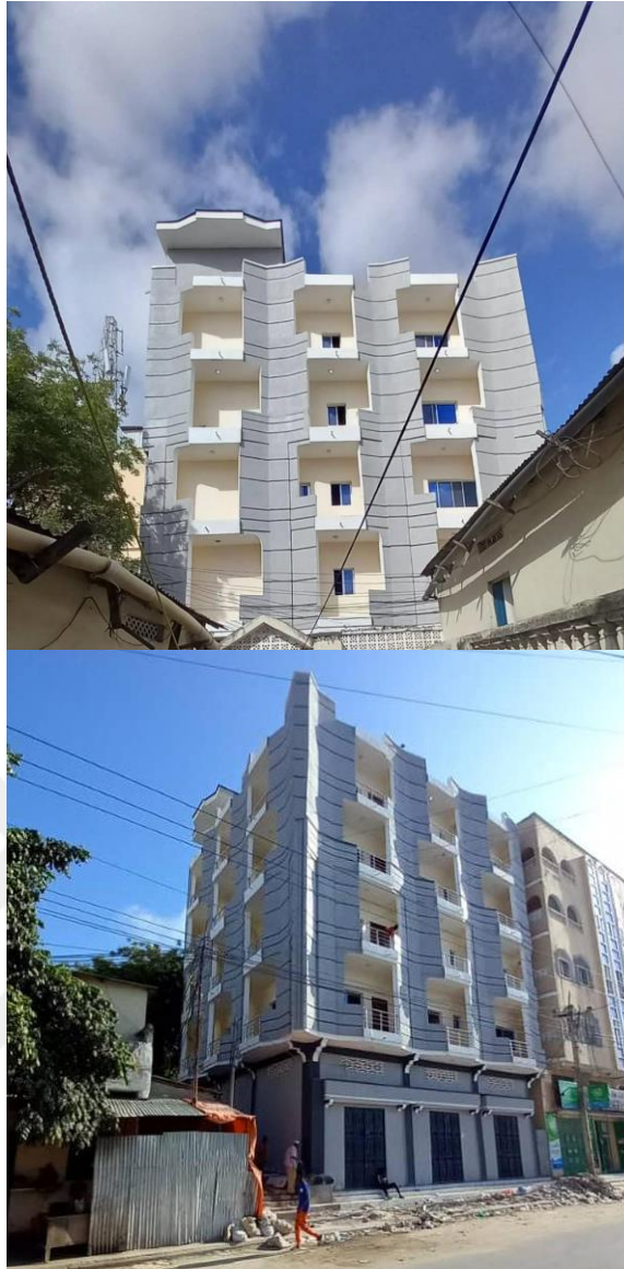
Figure 3.41: Renovated apartment (source owner)
