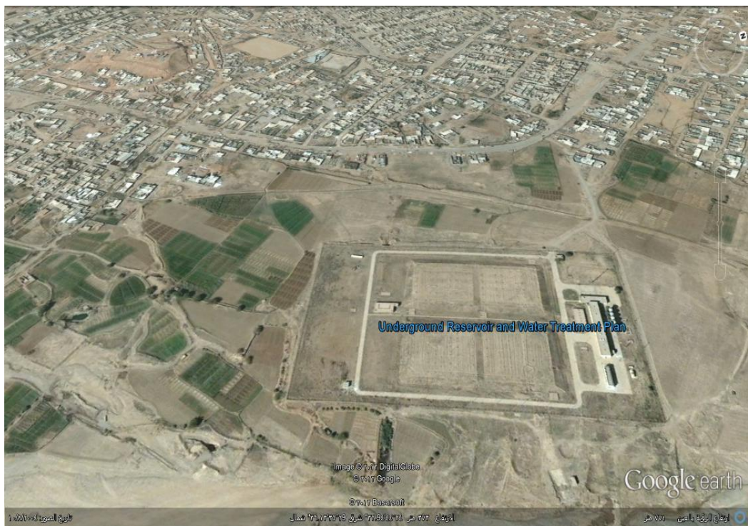
Figure 1.5 An underground Reservoir
