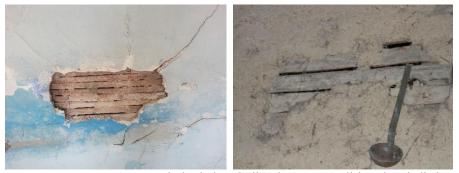
Figure 43. Examples of timber lathed "bağdadi" plaster at traditional Eğirdir houses
