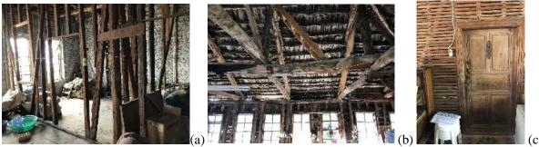
Figure 40. Traditional Eğirdir houses (a),(b) examples of timber framed system, (c) timber lathed "bağdadi"
