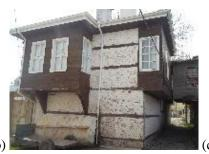
Figure 38. Construction system at traditional Eğirdir house (a) brick + stone masonry (b) stone masonry + timber framed (c) mixed use of systems.
