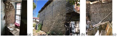
Figure 41. Wall fillings at traditional Eğirdir houses (a), brick filling (b), (c) adobe filling
