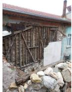
Figure 39. Using stone and timber framed system together in traditional Eğirdir houses
