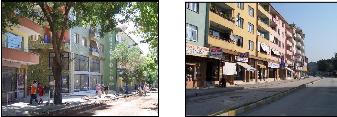
Figure 1 Trade Occupancy or Offices on the Ground Floor (Kirkkale and Düzce)
