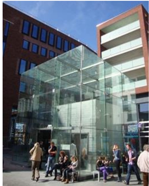
Fig. 1 Glass Cube in Haarlem's Raaks Square, built in 2011 and designed by Kraayvanger Urbis
