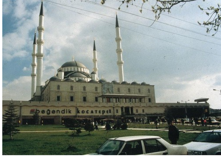
Figure 5.2: Beğendik Mall Situated on the Basement Floor of Kocatepe Mosque
