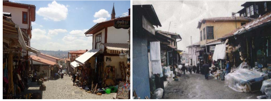
Figure 9. General view from Koyunpazarı Street (towards Ahi Elvan Mosque) (Karakuş, 2020; Uruk, 1998)
