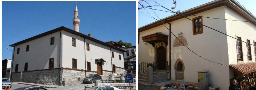
Figure 13. Ahi Elvan Mosque and Hacı Arap Mosque (Karakuş, 2020)
