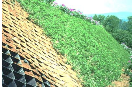
Figure 3.8. The Stages of Installing the Landscape Wall System (GEOsystems, 2014).
