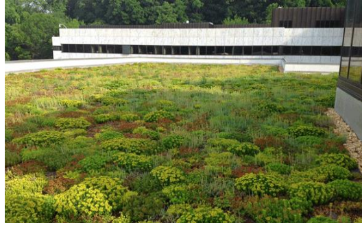
Figure 3.10. Semi-Intensive Green Roof (Furbish, 2015).
