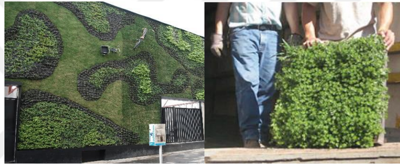
Figure 3.5. The Installation of Modular Living Wall That Has Been Grown Before (Timur & Karaca, 2013).
