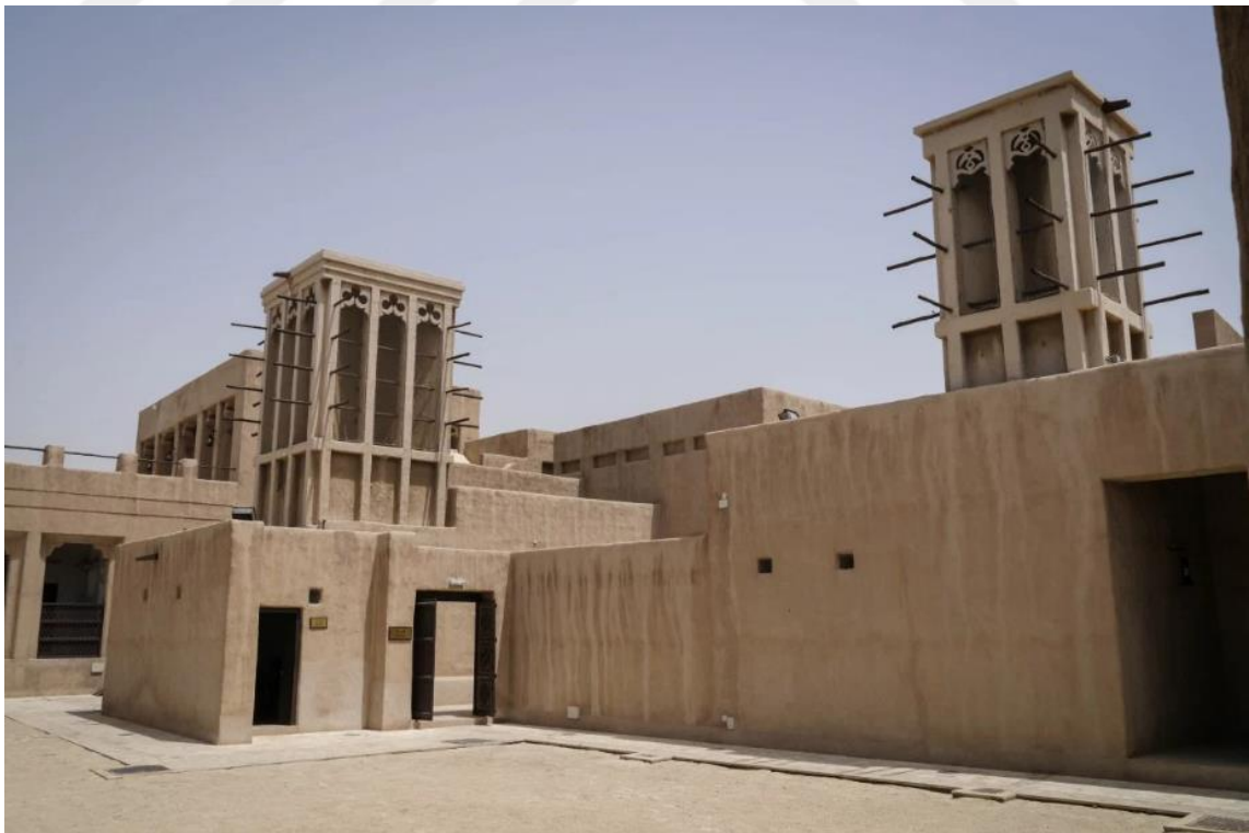
Figure 2.3: Wind towers for stack ventilation in ancient houses in the Arab Region (The City, 2013)
