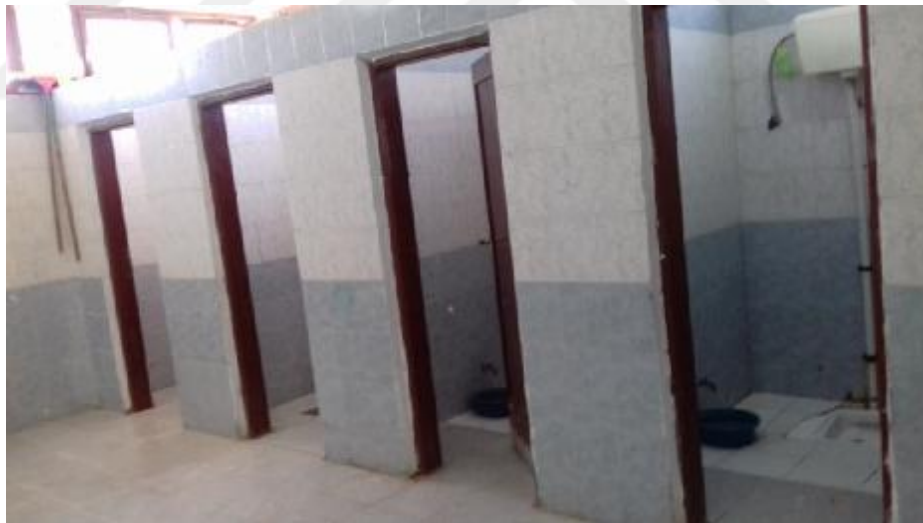
Toilets (Picture taken by author)
