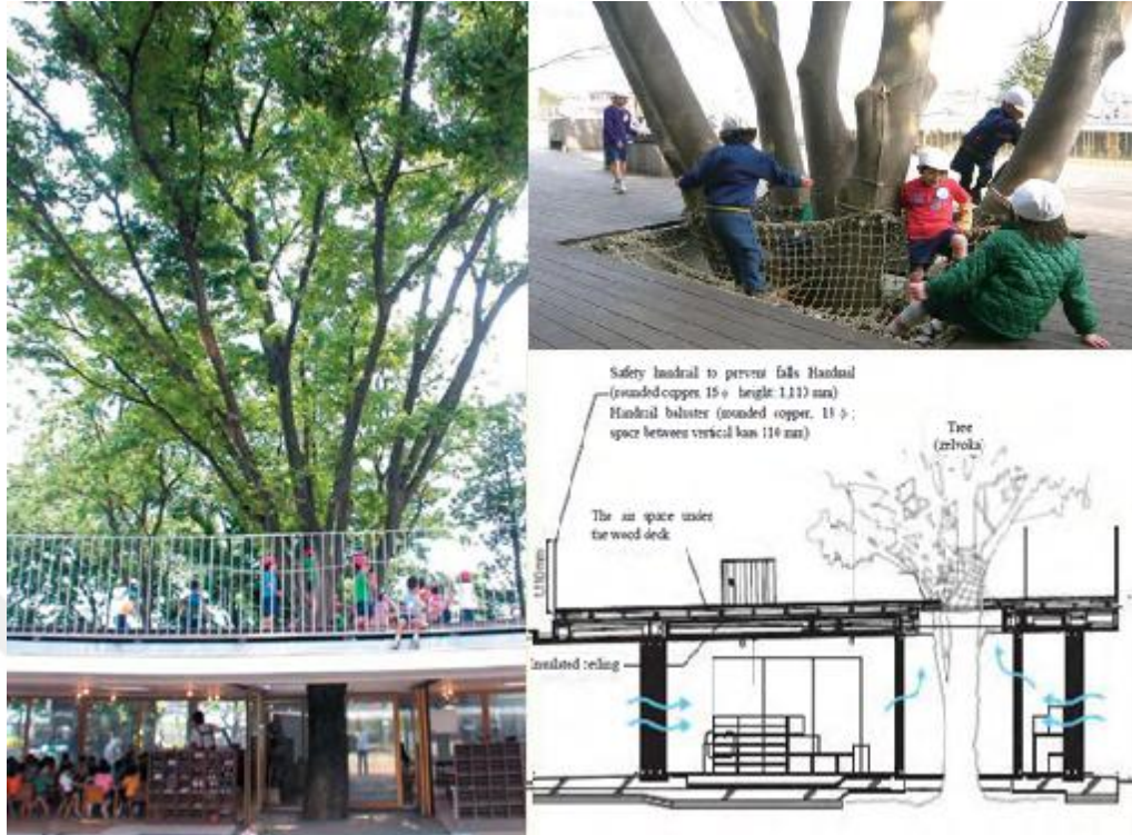
Figure 2.7: An environmentally friendly design of the rooftop at Fuji kindergarten, part of the playground, designed to sustain an existing tree and strengthen the children's tie with the environment (MECSST, 2010)
