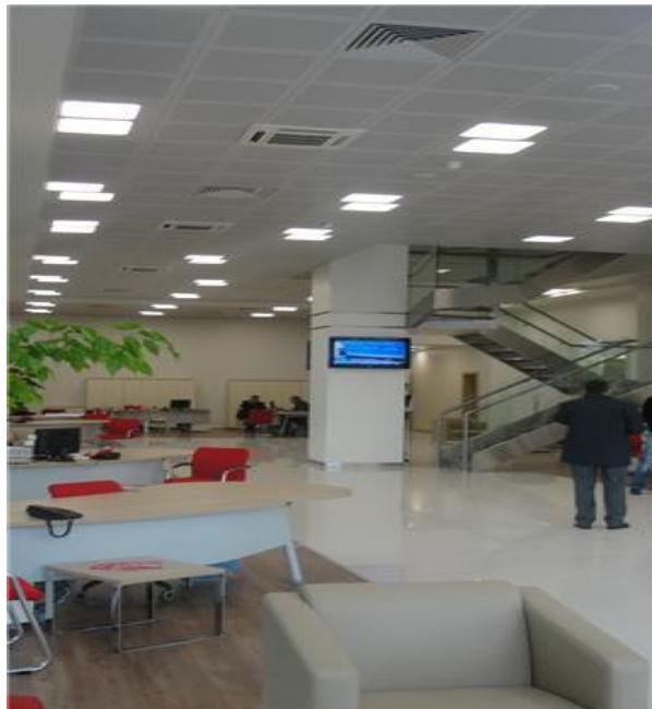
Figure 27: Ziraat Bank recessed lighting fixtures (taken by the architect of Ziraat Bank)
