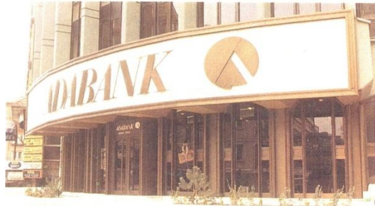
Figure 38: Adabank exterior facade
