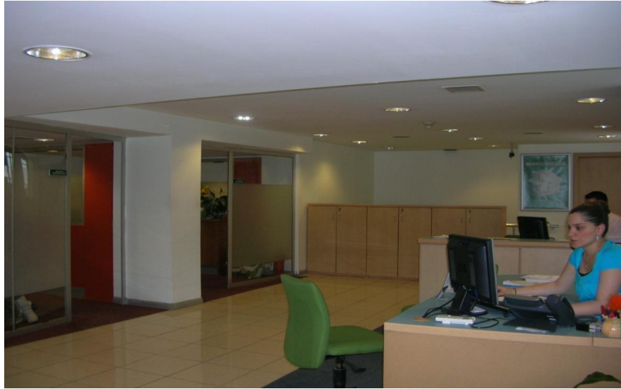
Figure 28: Garanti Bank recessed lighting fixtures in open office area (taken by the staff of Garanti Bank)
