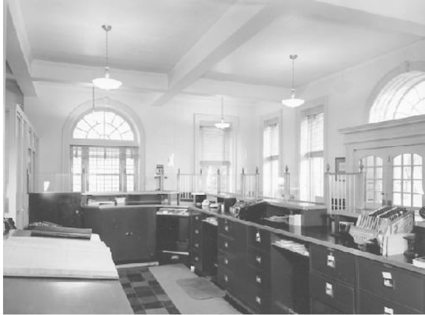
Figure 32: North Bennington Vermont Bank interior (photos are retrieved from www.google.com.tr/images )
