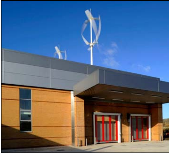
Figure 27: The Stores Building, Surrey, BREEAM Certificate, Excellent (BREEAM Certificated Projects, http://www.breeam.org/page.jsp?id=205 , 2010)
