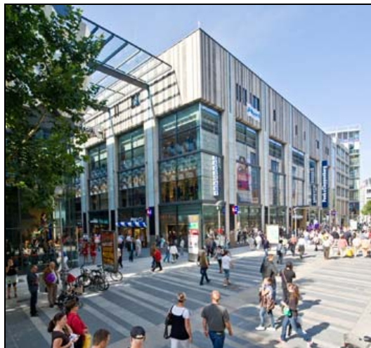
Figure 24: Centrum Galerie, Dresden, BREEAM Certificate, Excellent (BREEAM Certificated Projects, http://www.breeam.org/page.jsp?id=205 , 2010)
