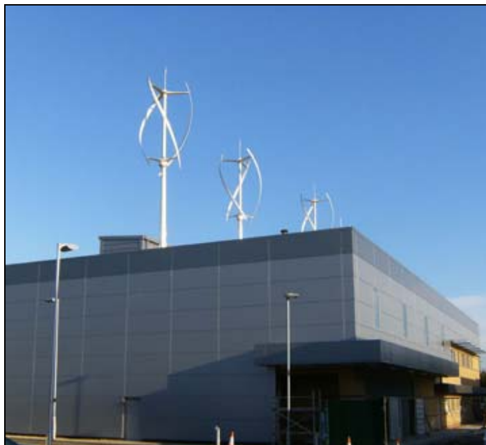
Figure 28: The Stores Building, Surrey, BREEAM Certificate, Excellent (BREEAM Certificated Projects, http://www.breeam.org/page.jsp?id=205 , 2010)
