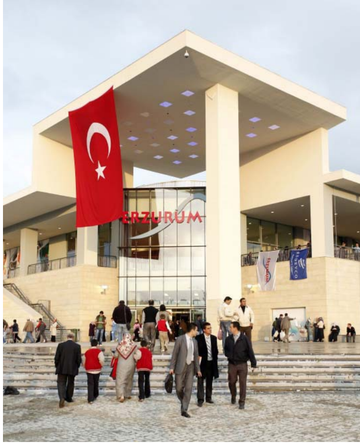
Figure 31: Erzurum Shopping Center, Erzurum BREEAM Certificate, Very Good (Yapı Dergisi, Ecology in Buildings, April 2010)
