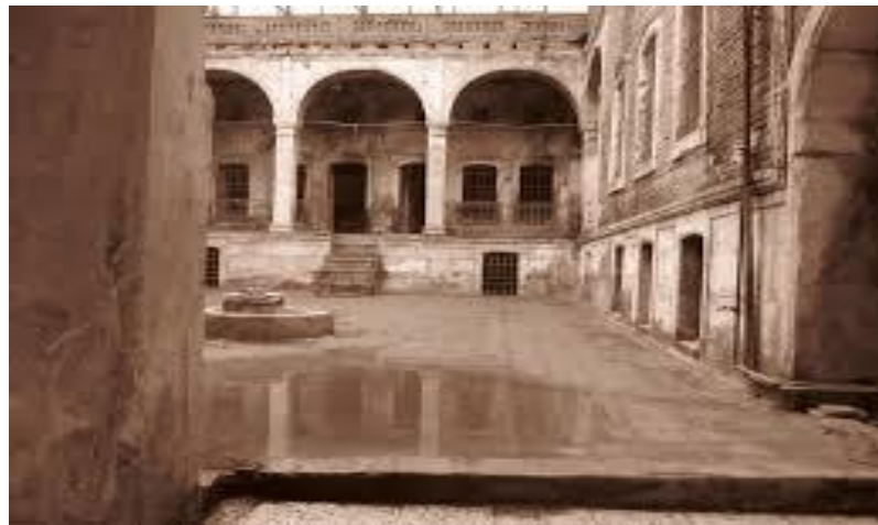
Figure 50 The Central Courtyard which has Lower Windows and Upper Windows to Let More Day Light [111]
