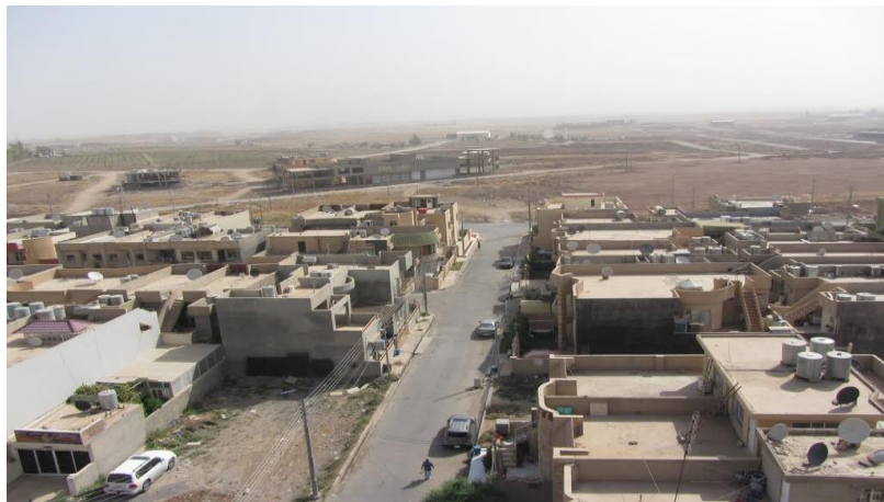
Figure 88 House in Modification Period- Erbil
