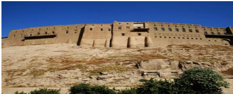
Figure 72 Erbil Citadel – Exterior Wall [77]
