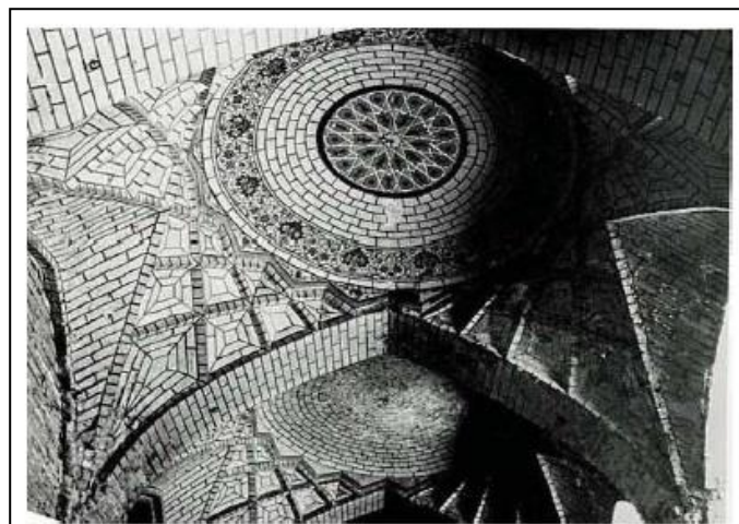
Figure 46 The Structure Material in the Basement is All Masonry [4]
