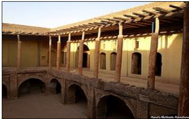
Figure 51 The Upper Floor Rooms with Wooden Columns (Colonnade, Tarma) and Surrounding the Lower Floor with Arcade [115]
