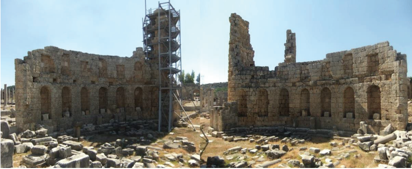
Figure 2. The South Gate of Perge (by the author)
