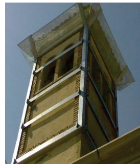
c) longitudinal and transversal ties
