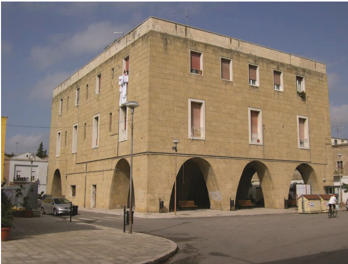
Figure 4. Incoronata (Foggia-Puglia-Italy) village, building of the municipality.
