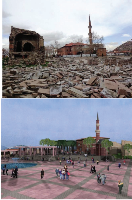
Figure 2. Arrangement of the Hacı Bayram Square Destroyed and Renewed at Mayor Melih Gokcek Period
