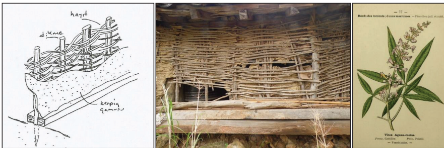
Figure 2. Left: perspective of the construction (drawn by author). Middle: detail photo of the bottom part. Right: Vitex agnus-castus locally called “Hayıt”
