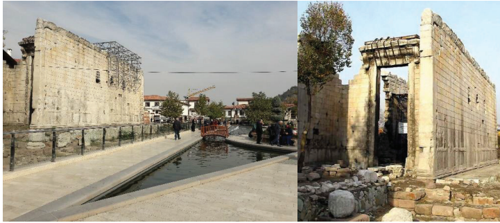
Figure 4. New pool and sitting places showing changing elements around Augustus Mosque.
