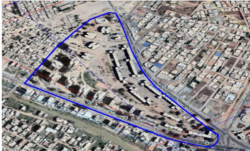
Figure 72: Lack of Parks and Children's Playgrounds
