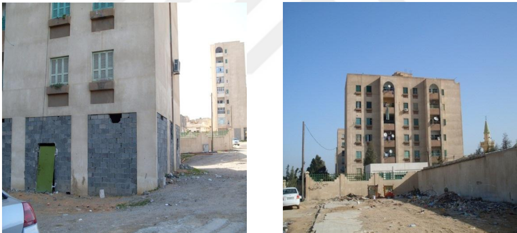
Figure 49: Some Photos for the Site AirPort Housing Project
