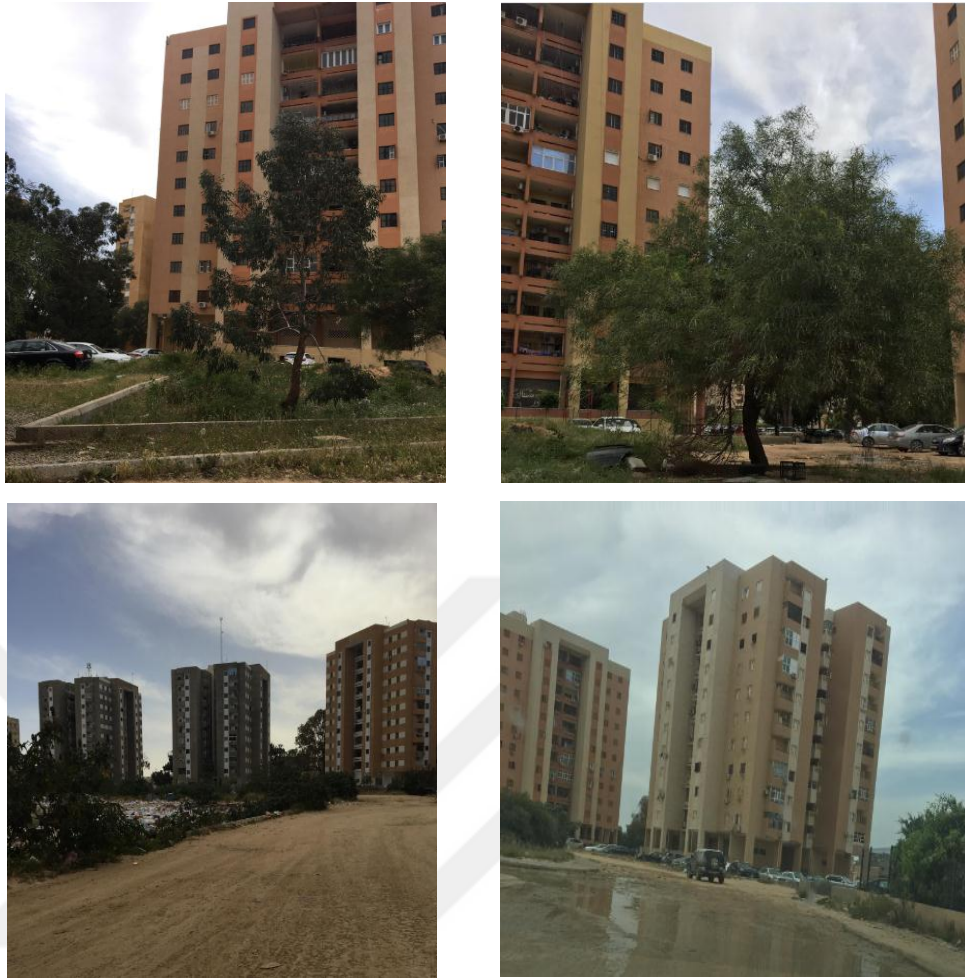
Figure 54: Incomplete Environment (Garden, Pathways & Access Streets)
