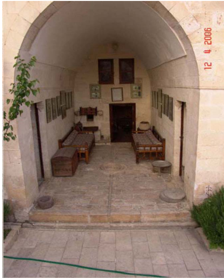
Picture 4.2.9 Cooling Space (Mungan House)
