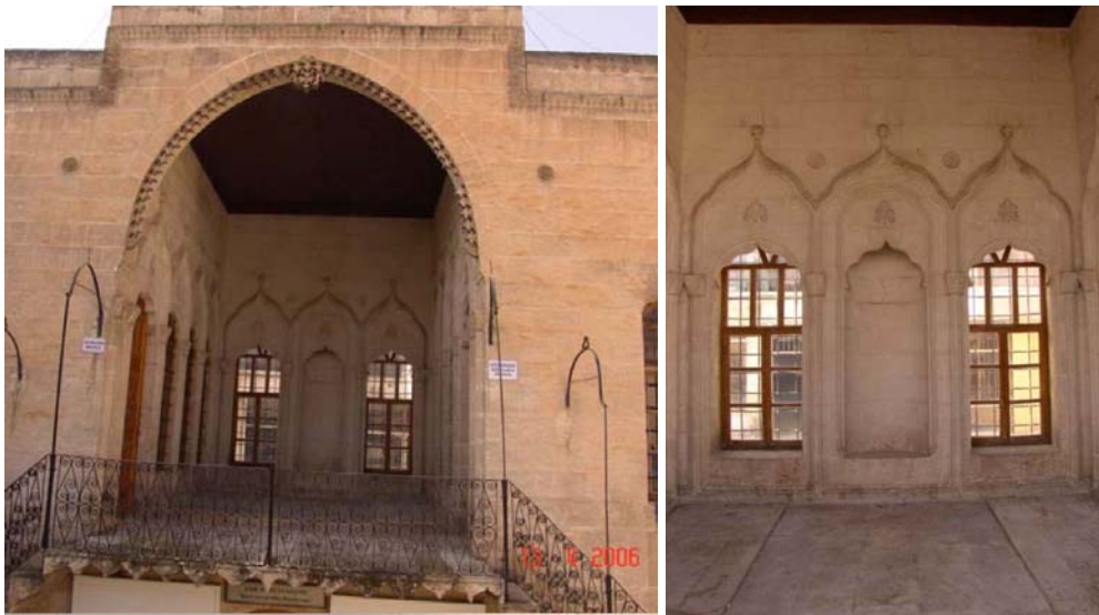
Picture 4.2.8 Mungan House, Eyvan of Semi Open Space
