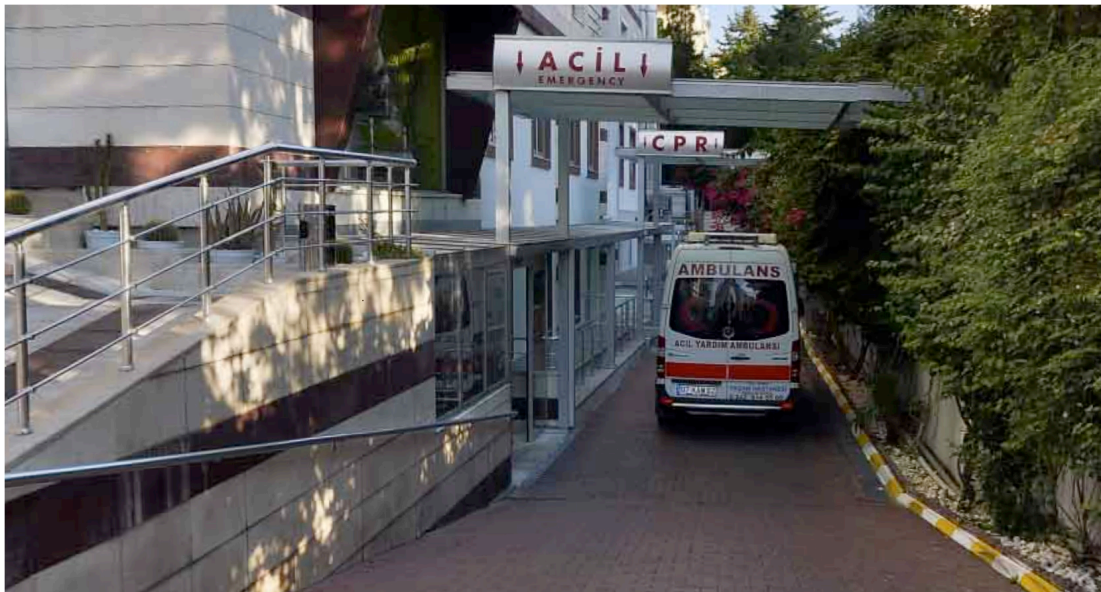
Figure 10. Emergency service entrance of sample A (photo taken by the author)
