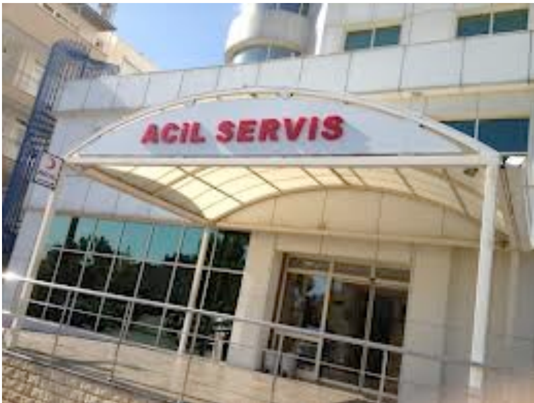
Figure 15. Emergency service entrance of sample B
