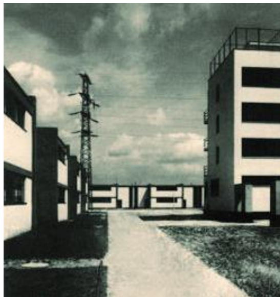
Figure 4. The Toerten houses in Germany (1926-28) is one of the first examples of industrialized building block buildings. [30]
