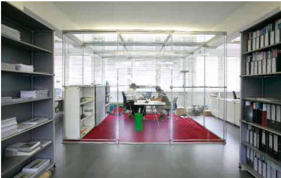
Figure 20. Meeting room divided from open plan offices with the system of terminal as partitions. [86]
