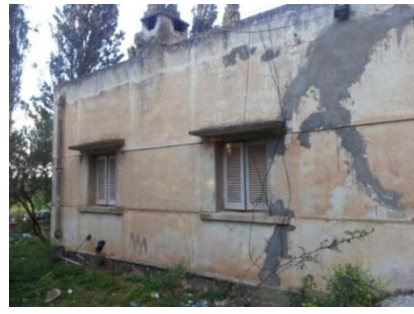
Figure 38. Shows the rear of the house to the presence of windows and heating nozzle
