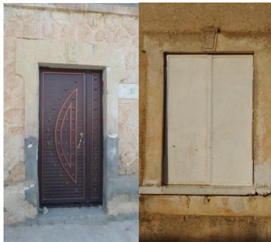
Figure 26. Door and window of the house there is a change in the door just shows
