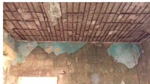
Figure 69. Showing the house roof and show the materials used
