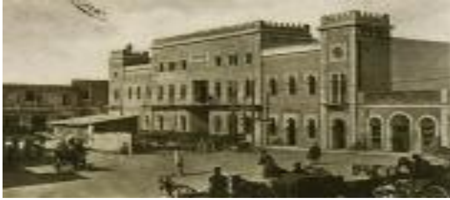
Figure 4. Municipality Benghazi building
