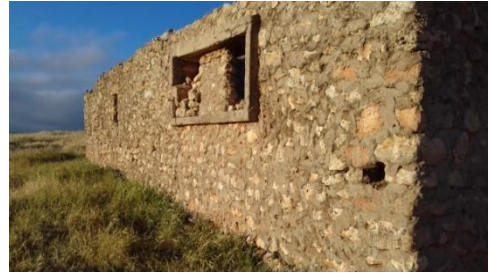
Figure 79. Showing the left side of the house
