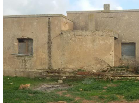
Figure 72. Showing the back of the house from the windows without a change in the Italian style
