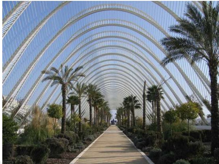
Figure 48. L'Umbracle by Santiago Calatrava's. (Url 40)
