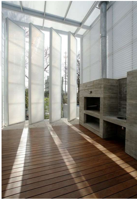
Figure 41. The Movable Panels are Composed by a Double Skin of Rough Polycarbonate. (Url 34)
