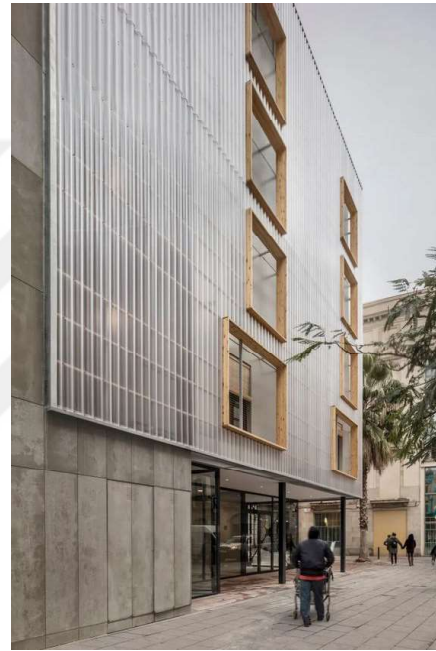
Figure 42. Façade Design with Polycarbonate Material. (Url 35)
