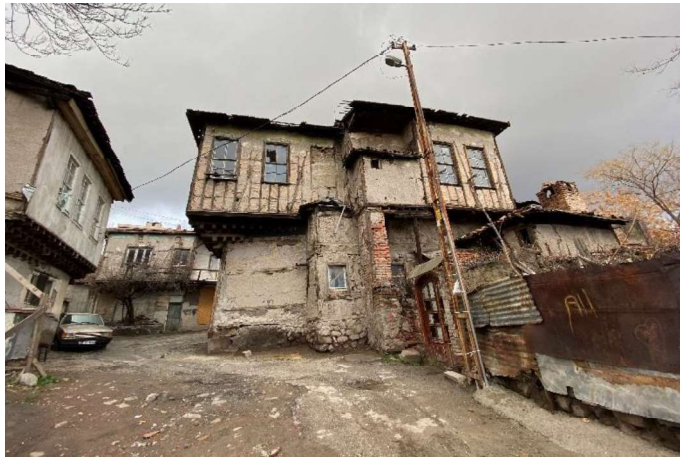
Figure 62. Streets in Ruins in the Hamamarkası Region (Author's Archive, 2021)
