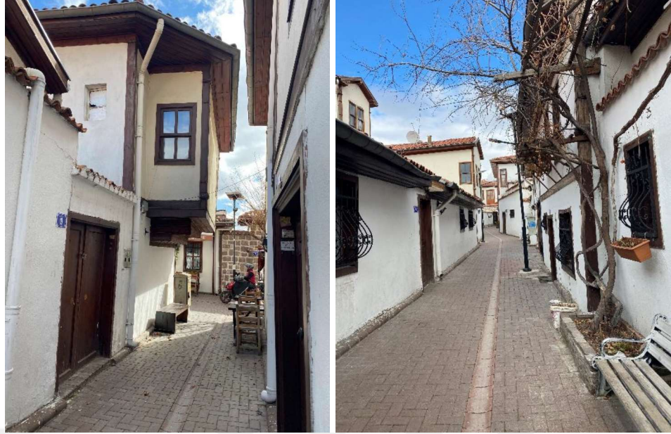
Figure 61. Hamamönü Region, Fırın Street Street Rehabilitation Project Implementation (Author's Archive, 2021)
