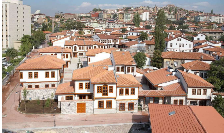
Figure 91. A Section of Hamamönü Region in 2012 (Altındağ Municipality, 2014)
