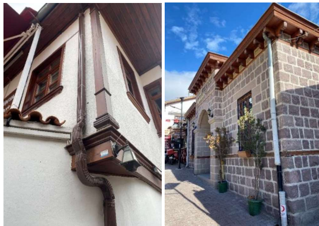
Figure 109. Façade Pipes, 2021 (Author's Archive)
