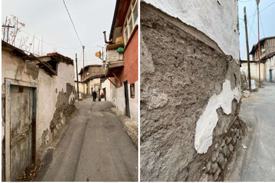
Figure 41. Hamamönü Region, Ankara House In Ruins Stone Material, Courtyard Door, Street Buildings (Author's Archive, 2021)
