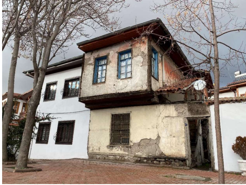
Figure 24. Hamamarkası Region, New and Old Buildings Side By Side Bay Window, Eaves, Stone Floor, Tile Cover, Window Iron Railing (Author's Archive, 2021)
