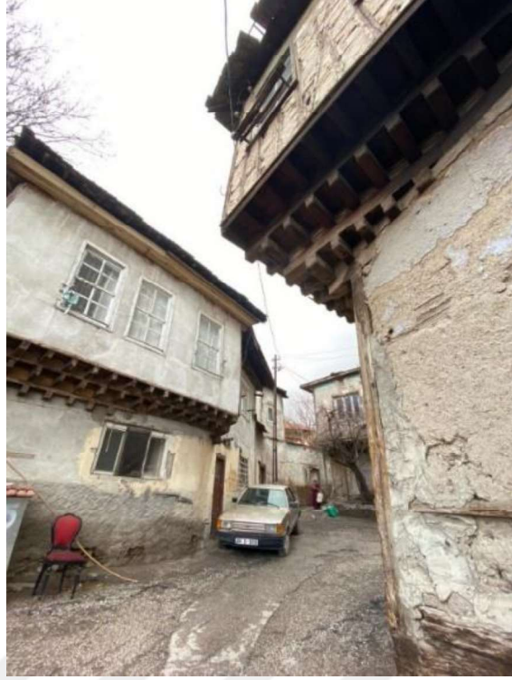
Figure 44. Traditional Ankara Houses, 3-Step Corbelling Projection Examples Hamamarkası Houses (Author's Archive, 2021)
