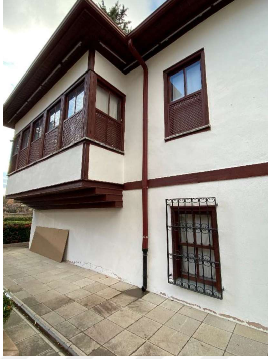
Figure 48. Hamamönü Region, Mehmet Akif Ersoy House Museum Street Rehabilitation Project Implementation Wood Lattice, (Author's Archive, 2021)
