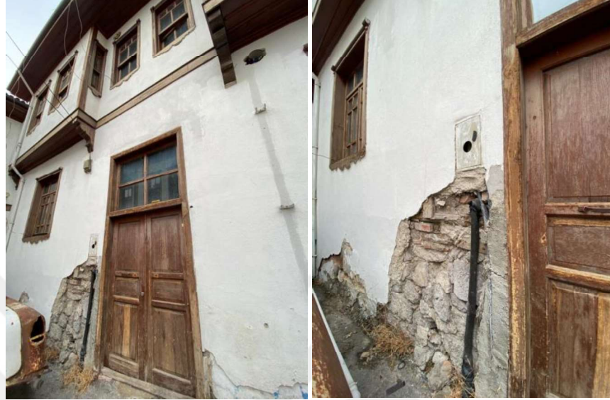
Figure 39. Hamamönü Region, Ankara House Stone Material, Simple Console Projection, Windows, Eaves, Entrance Door and Top Window (Author's Archive, 2021)
