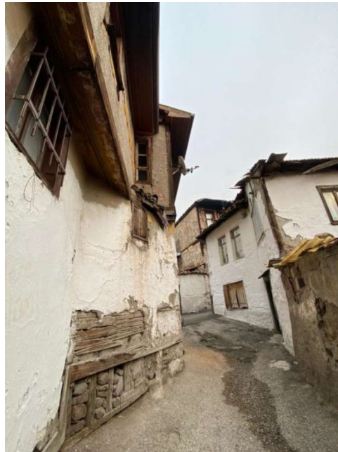
Figure 40. Hamamönü Region, Ankara House Stone Material, Railing, Projection, Eaves, Street Buildings (Author's Archive, 2021)
