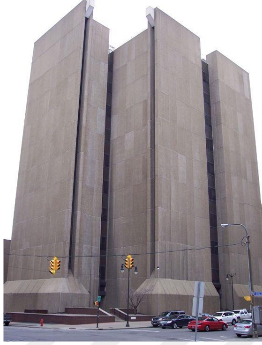
Şekil 3. 23: Buffalo City Court Building (url-16)
