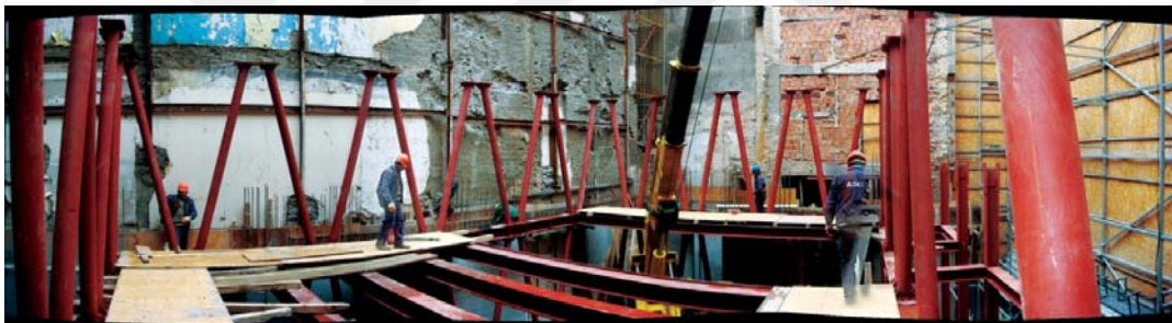
Figure 5.1 Photographs of the construction phase as taken by GAD (GAD, February 2008)
