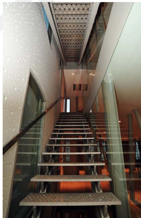
Figure 5.32 New steel stairs
