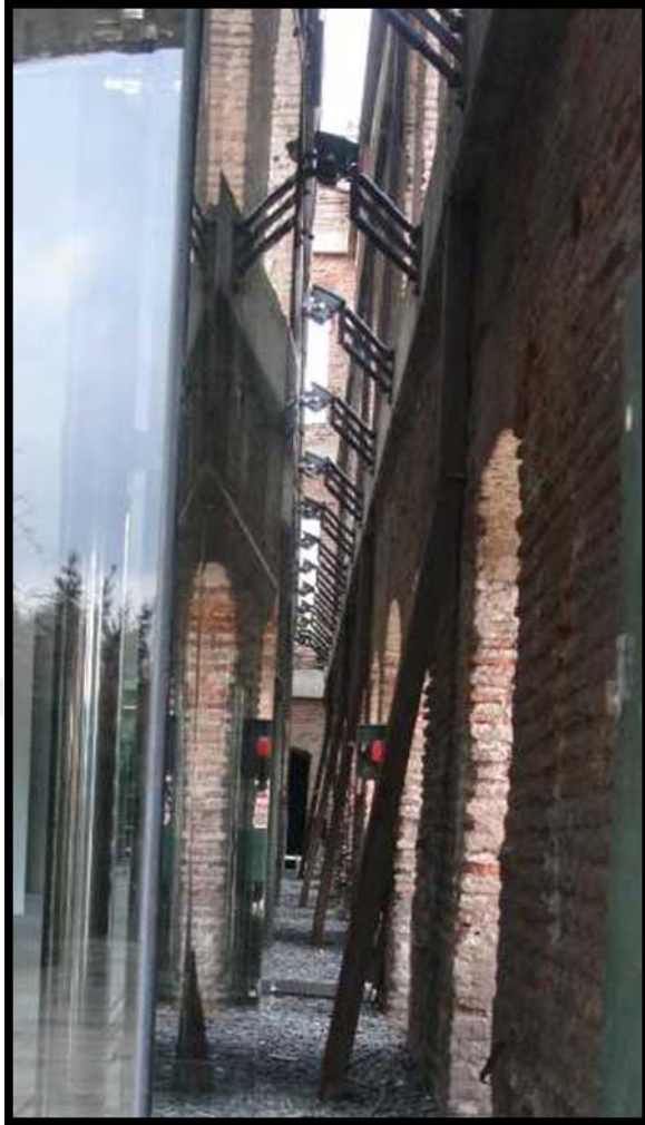
Figure 3.18 Combination of old brick facade and new steel structure
