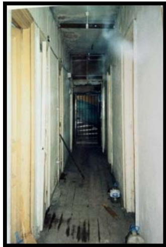
Figure 4.30 Hanging light in the ceiling, wooden floor on ground
