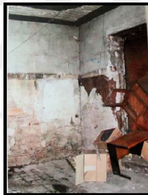
Figure 4.33 Masonry bricks can be seen on walls
