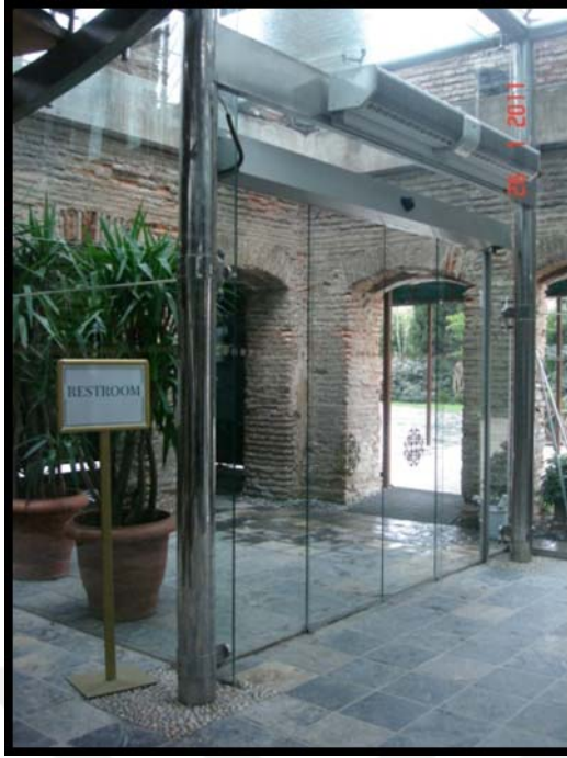
Figure 3.11 Main entrance (photorecell sliding glass door)
