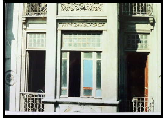
Figure 4.11 French balcony of 2 nd floor
