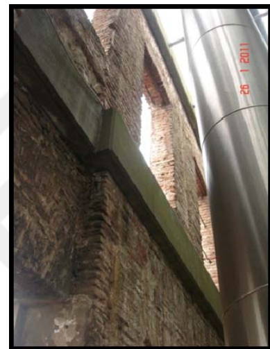
Figure 3.20 Retrofit reinforced concrete brace or wrapping
