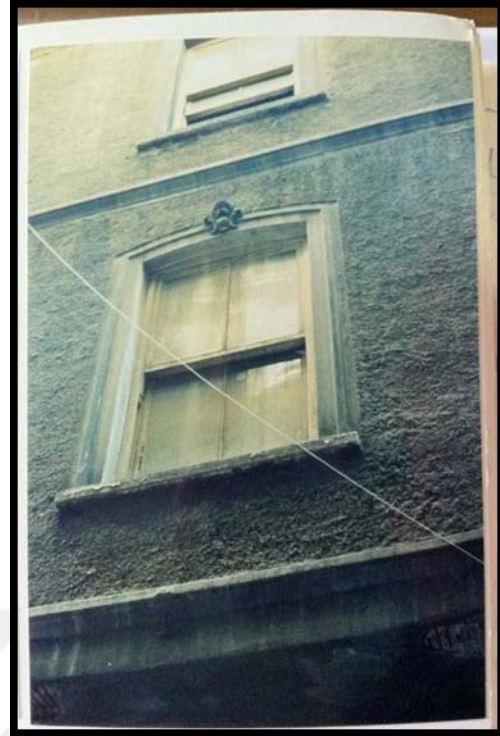
Figure 4.17 Windows of facade facing OS
