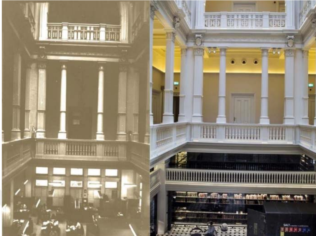
Figure 3.50 Courtyard old new
