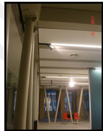
Figure 4.66 Ceiling and lighting on first floor
