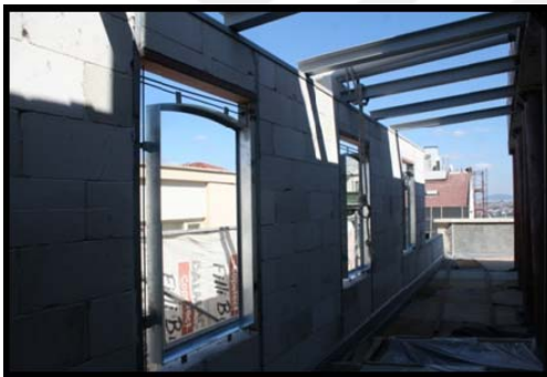
Figure 4.52 Four openable joineries for terrace construction photo
