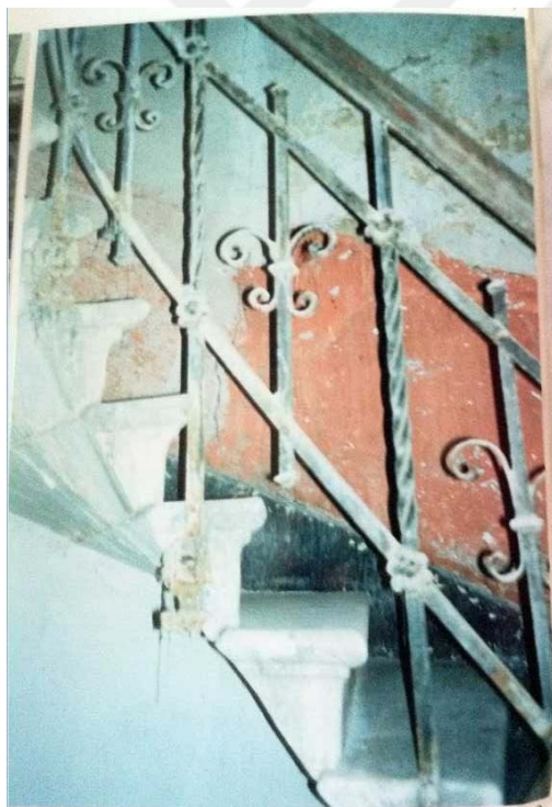
Figure 5.31 Old concrete stairs
