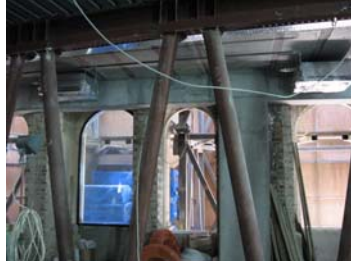
Figure 5.7 Air conditioners were mounted on ceiling (GAD, August, 2008)
