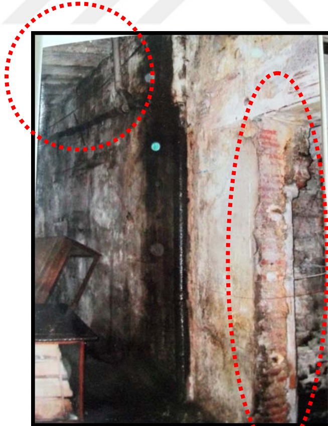
Figure 4.20 Ceilings of ground floor and walls are masonry brick
