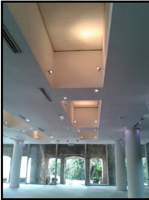
Figure 3.13 Ground floor rear window door and suspended ceiling
