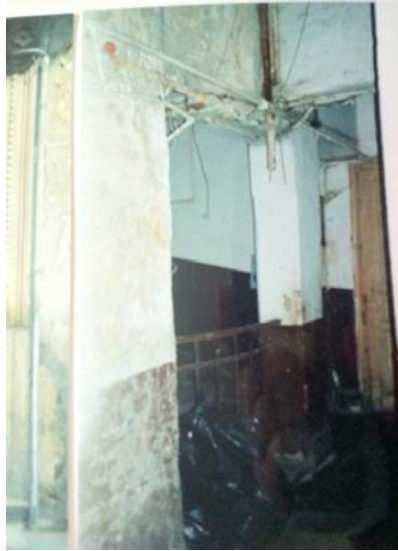
Figure 5.27 Old structural system, concrete column
