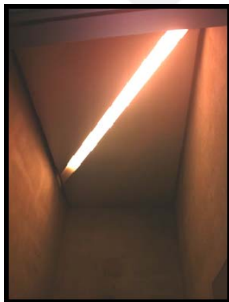
Figure 4.69 Restroom ceiling lighting
