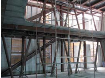
Figure 5.6 Scaffolding in gallery space (GAD, August, 2008)
