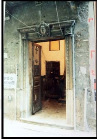
Figure 4.13 Ground floor facade facing OS door
