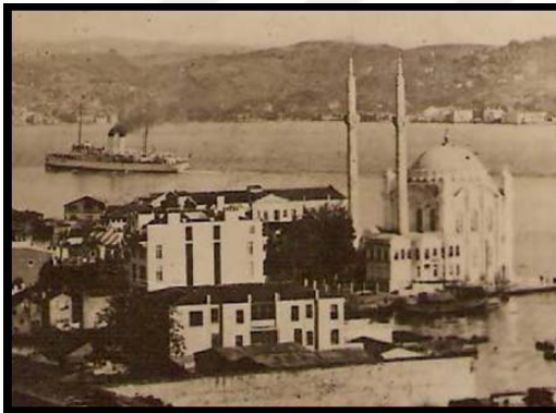
Figure 3.1 Roofed ESM before construction of Bosphorus Bridge
