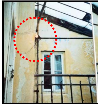
Figure 4.31 Natural light is taken from skylight
