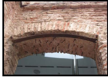
Figure 3.19 Belt reinforcement
