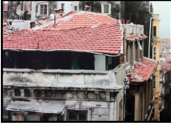
Figure 4.35 Marseille roofing tile has been used in roof. The roof is in the form of hipped roof
