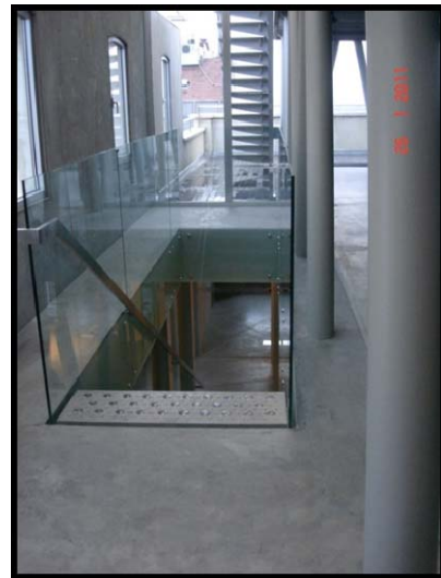
Figure 4.53 Photo of completed form of 4 openable joineries for terrace
