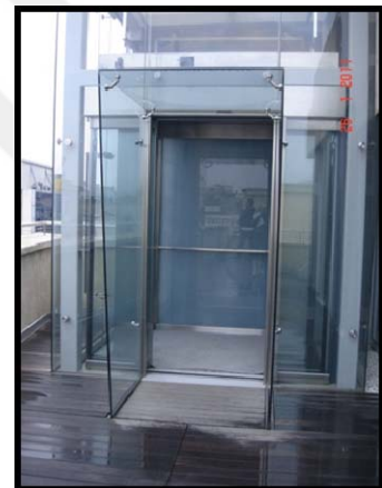
Figure 4.71 Elevator door at terrace floor
