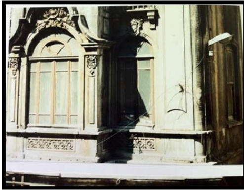
Figure 4.10 Stone archs of 1 st floor
