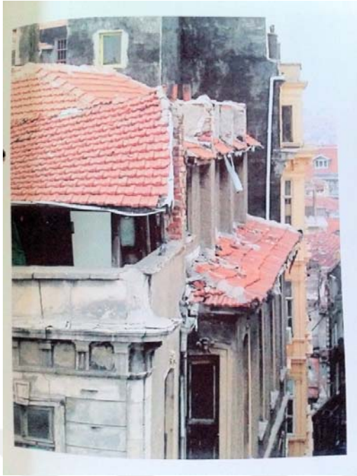
Figure 5.29 Roof floor old structural system, tile roof
