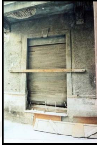
Figure 4.14 Ground floor facade facing OS window
