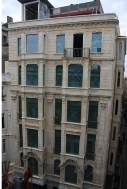
Figure 5.12 Outer windows of the building were installed (GAD, November 2008)
