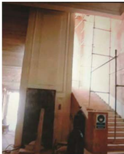
Figure 3.55 Elevator used in the Ottoman Bank [28]
