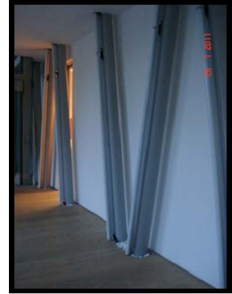
Figure 4.46 Corridor on the 4 th floor
