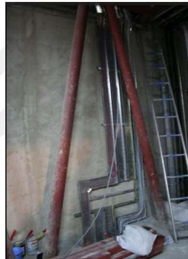
Figure 5.11 Electricity and installation pipes were installed in the shafts (GAD, September 2008)
