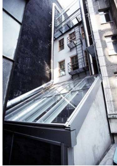
Figure 3.34 Changa Restaurant's new rear facade
