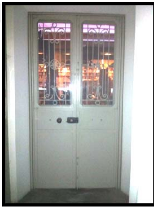
Figure 4.37 Fire exit door at ground floor
