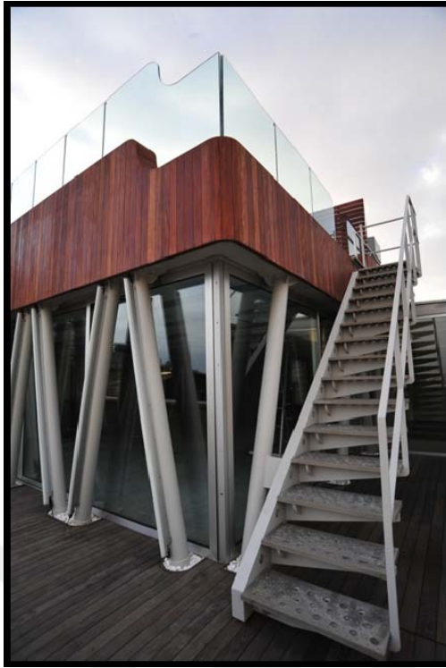
Figure 4.47 Stairs from terrace to roof
