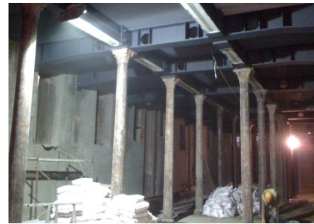
Figure 3.48 Construction work on the Forum area
