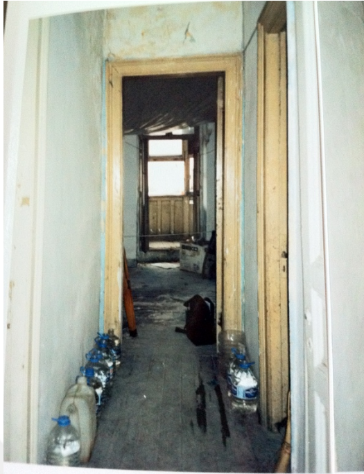
Figure 5.24 Old fifth floor corridor and balcony
