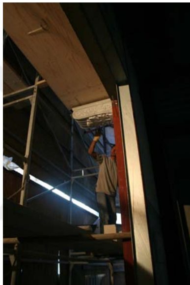
Figure 5.10 Original front facade was restored (GAD, September 2008)
