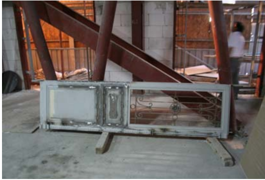
Figure 5.9 Original side door was restored in situ (GAD, September 2008)
