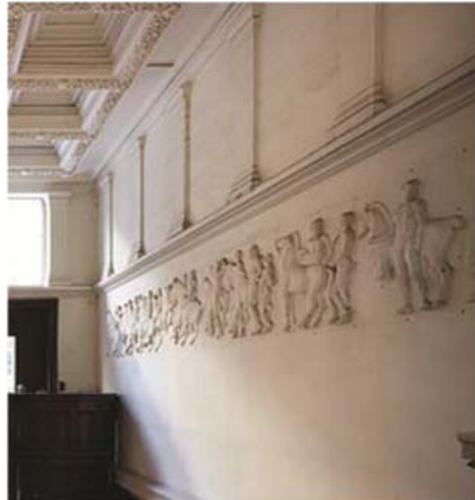
Figure 3.53 Ottoman Bank entry wall [28]
