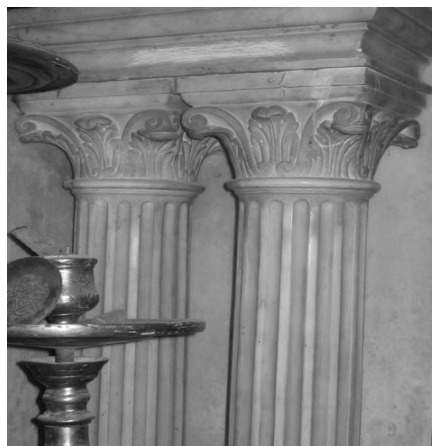
Figure 4.36 Marble Columns with Corinthian Capitals of Mihrab of M. Gurgi Mosque 1833-1838 (Samira.N.B.Said. 2005)
