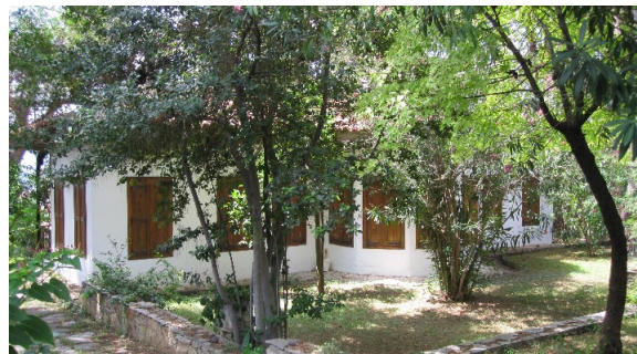
Figure 15. Northern facade of Nail Cakirhan House. Photograph by the author.
