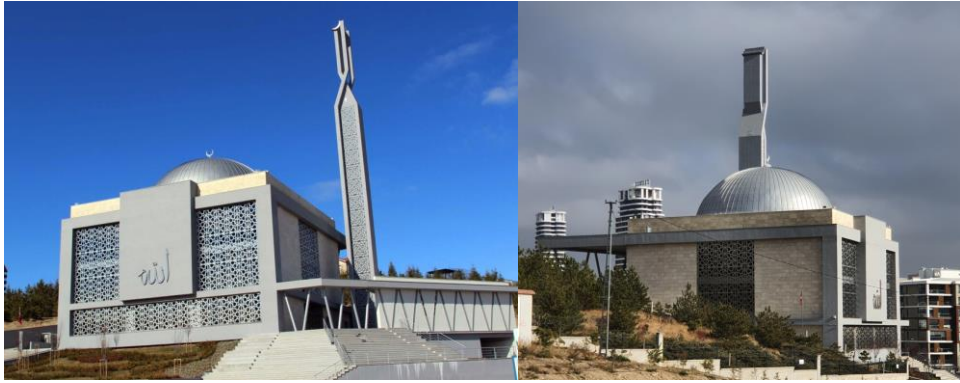
Fig. 6 - Looking at Uluyol Mosque from southeast and southwest directions
