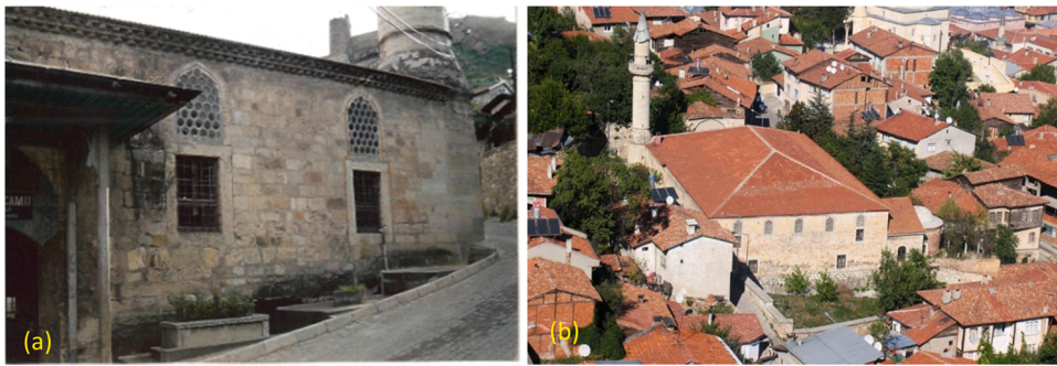
Fig. 1. The views of the mosque before the restoration. (a) Entrance, (b) Perspective.
