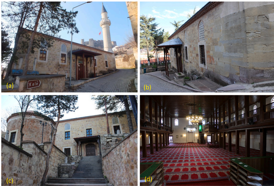
Fig. 4. Post-restoration images of the mosque. (a-c) Two entrances of the mosque (d) Interior of the mosque.
