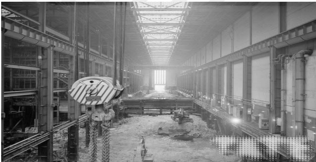
Figure 17: Excavating the Turbine Hall Bankside Power Station 1996 (URL 13).
