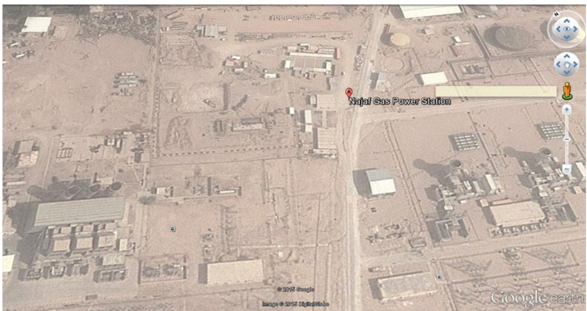
Figure 15 Satellite Image of Al Najaf Power Plant
