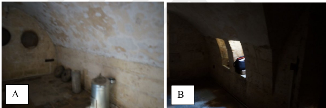
Figure 49: B1 Room Photos (A,B) (Photo by Author)
