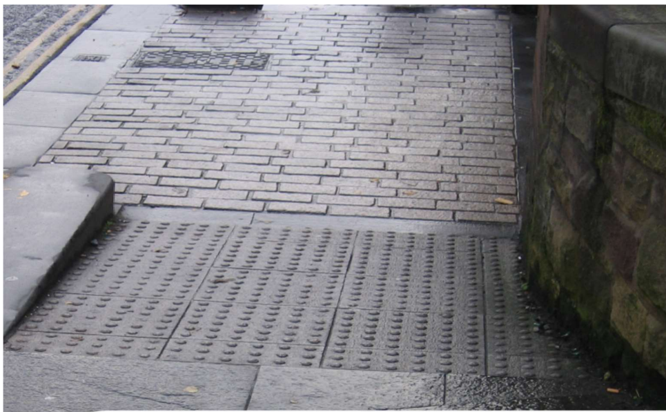
4.4. Tactile paving design guide 003
