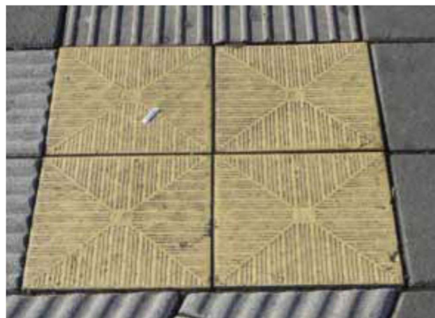
4.1.19. Netherlands-Style Warning Blocks(Amsterdam, Netherlands)
