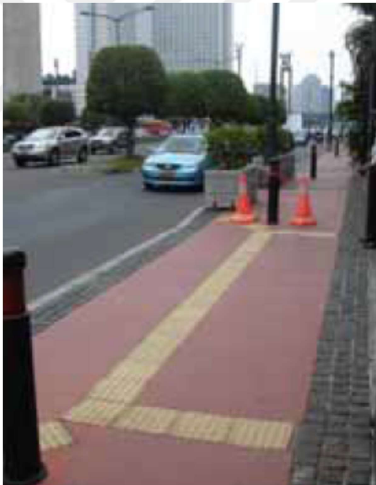
4.3.5. Tactile Ground Surface Indicators Used to Indicate Parking Lot Entrances (Jakarta, Indonesia)
