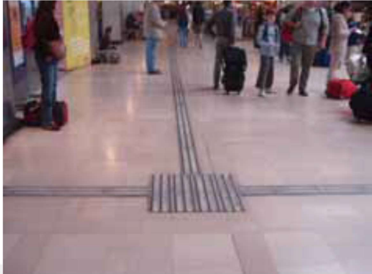
4.1.11. Tactile Ground Surface Indicators at Montparnasse Station (Paris, France)
