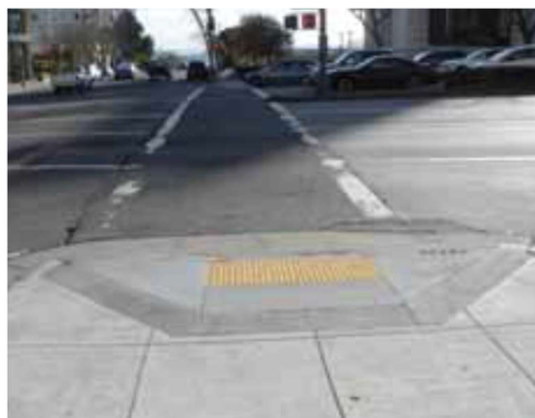
4.2.2. Tactile Ground Surface Indicators before a Crosswalk (San Francisco, USA)
