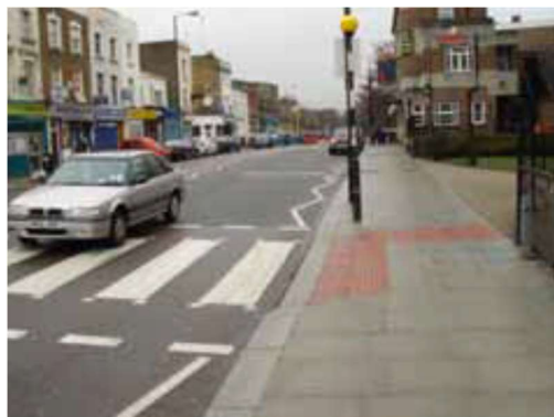
4.1.1. L-Shaped Tactile ground surface indicator Installation (London, UK)
