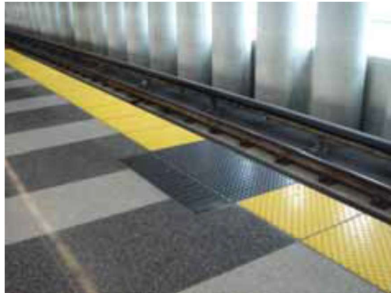
4.2.3. Tactile Ground Surface Indicators at a Rail Station Platform (San Francisco, USA)
