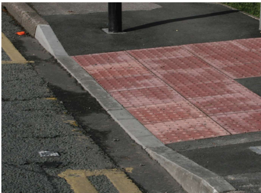
4.3. Tactile paving design guide 003
